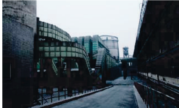
The Meishan wastewater treatment plant collected waste water from 12 industrial parks. Water quality is to be controlled and analysed continuously.
